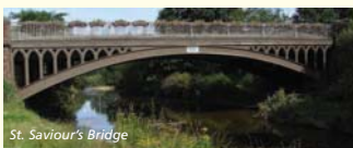
St. Saviour's Bridge
